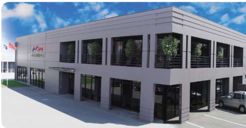
AuCom manufacturing plant in Christchurch, New Zealand.
